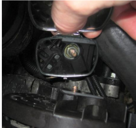
12V Lead removed
